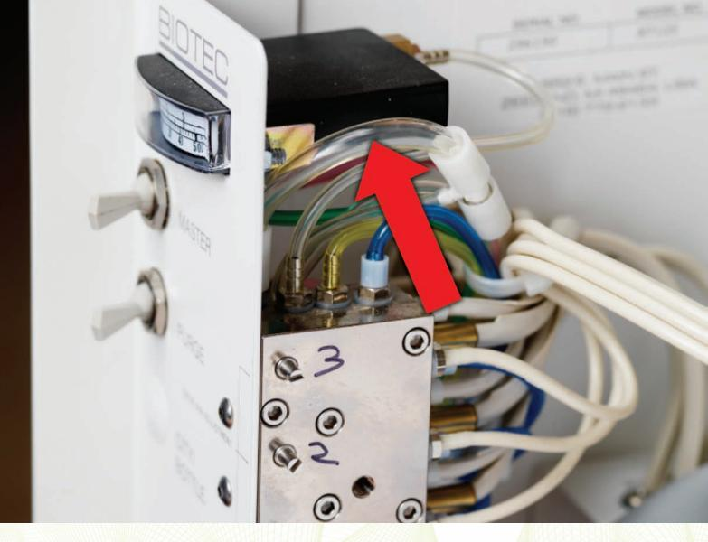
Biotec N7125 Connecting the Controller Main Air | Mounting the Controller | Installation Tips
